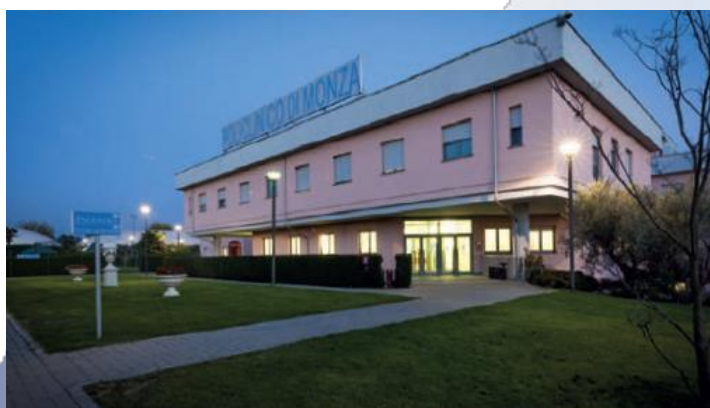
Entrance to the structure
